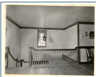
VIEW FROM SECOND FLOOR LOUNGE LOOKING NORTH TOWARD STAIR LANDING AND HANDRAILING OF STAIRWELL.
