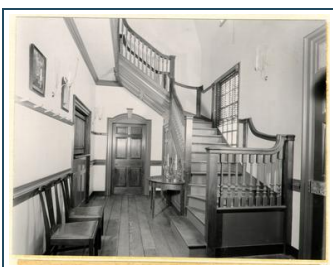
MAIN STAIRCASE IN ENTRANCE HALL OF KING'S ARMS TAVERN, LOOKING WEST. THE BAR IS VISIBLE AT REAR, LEFT. THE DOORWAY NEARBY LEADS TO NORTHWEST DINING ROOM.
