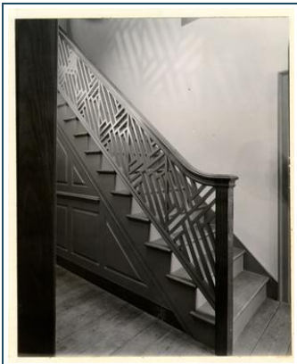
CHINESE CHIPPENDALE RAILING OF REAR STAIR OF KING'S ARMS TAVERN
