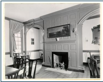
DINING ROOM (#2) OF TAVERN WING: FIRST FLOOR, LOOKING SOUTHEAST TOWARD FIREPLACE AND ARCHED DINING ALCOVES.
