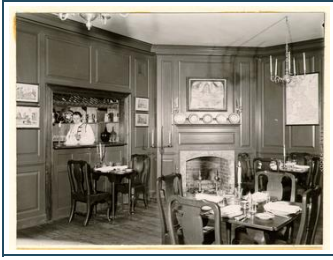
NORTHWEST DINING ROOM (#1), FIRST FLOOR, OF KING'S ARMS TAVERN, LOOKING SOUTHEAST TOWARD BAR AND FIREPLACE.
