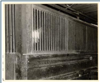
OLD BAR WITH SWINGING GRILLE IN BASEMENT OF PRINTING OFFICE IN MADISON, VA. IN THIS PICTURE THE GRILLE IS SHOWN IN THE CLOSED POSITION.
