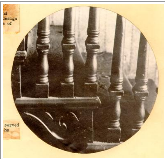
Balusters of LIBERTY HALL* served as model for balusters of the Anderson House stairway.
