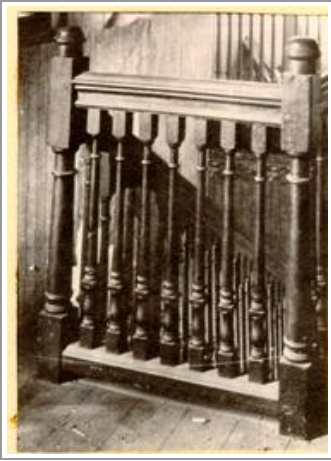
Stair Railing of LIBERTY HALL, at Second Floor.
