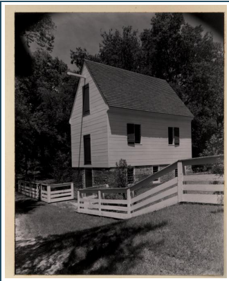
SOMEWHAT MORE DISTANT VIEW OF THE STOREHOUSE AFTER ITS RESTORATION, SHOWING THE SAME TWO SIDES OF THE BUILDING. THE FRAME SUPERSTRUCTURE WAS REBUILT ON THE BASIS OF EXISTING DOCUMENTARY AND PICTORAL EVIDENCE AS TO THE APPEARANCE OF THE OLD BUILDING.
