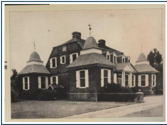
MULBERRY, AN OLD PLANTATION HOUSE ALONG THE WEST BRANCH OF THE COOPER RIVER IN SOUTH CAROLINA. THIS HAS A VESTIGIAL MEDIEVAL TOWER AT EACH OF THE FOUR CORNERS, THE TOP OF WHICH HAS A ROOF SIMILAR IN FORM TO THAT OF THE OFFICE.
